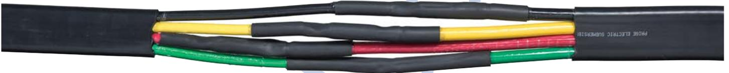
3rd Step: Apply Heat Shrink over butt splice and self-vulcanizing rubber tape.
