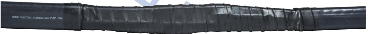
4th Step: Apply self-vulcanizing rubber tape over all exposed cables.
